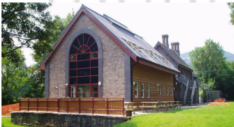
*Talybont is owned and maintained by Newport CC Address: The Old Station, Station Road, Talybont on Usk, Powys LD3 7YP
